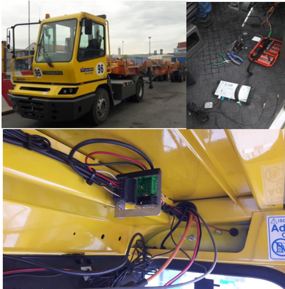
Figure 151: LL Koper - UC5 - Installing Telemetry IoT devices in Port Terminal Trucks.
