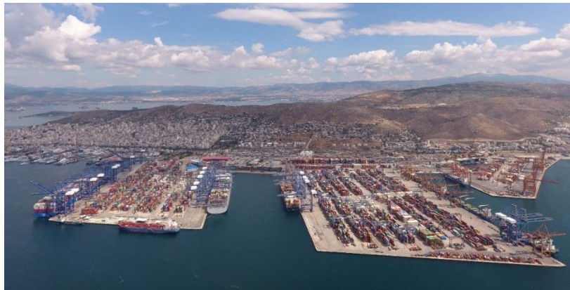
Figure 3: Athens Living Lab: port overview
