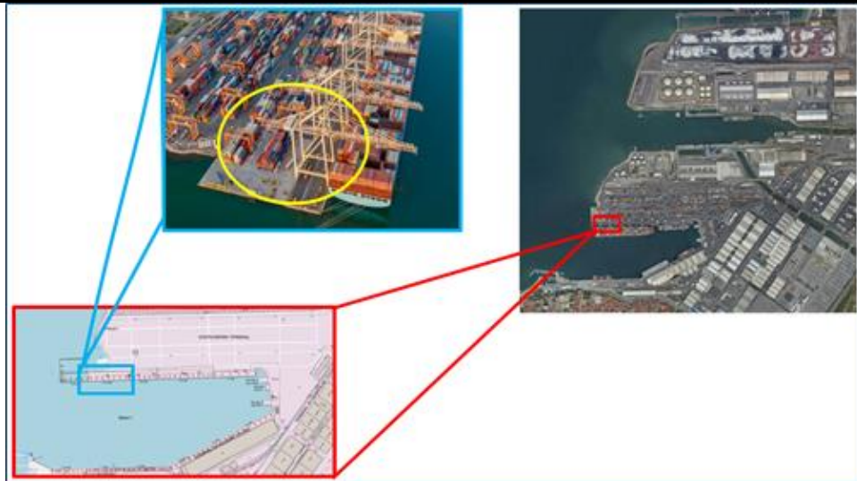
Figure 90: Port of Koper - Pier I: Location of STS crane KD 60
