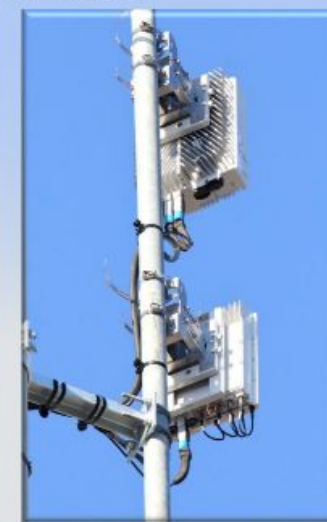
4G mRRH & 5G mmW Active Antenna already installed on a new pole, back side
