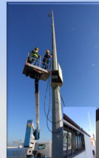
Crane elevator on the DC & optic fiber cabling installation working
