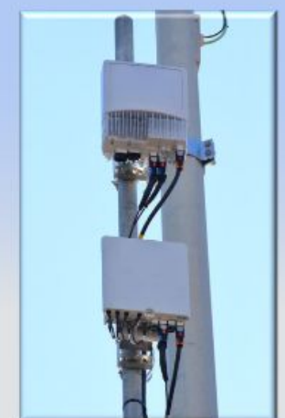
4G mRRH & 5G mmW Active Antenna already installed, front side
